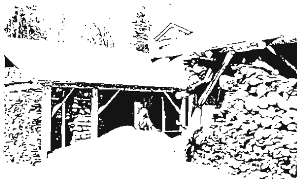
Figure 4. Open-sided wood storage.
